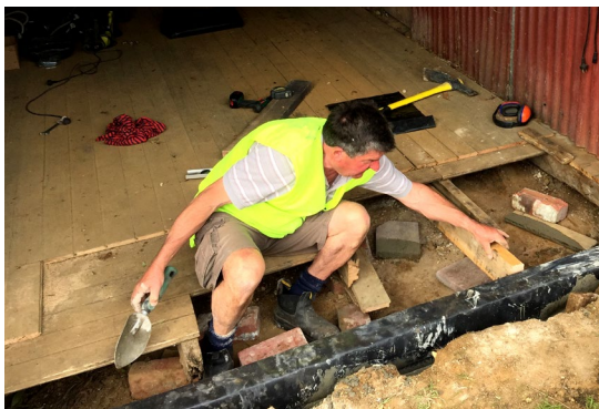
Peter working on the barracks floor.
